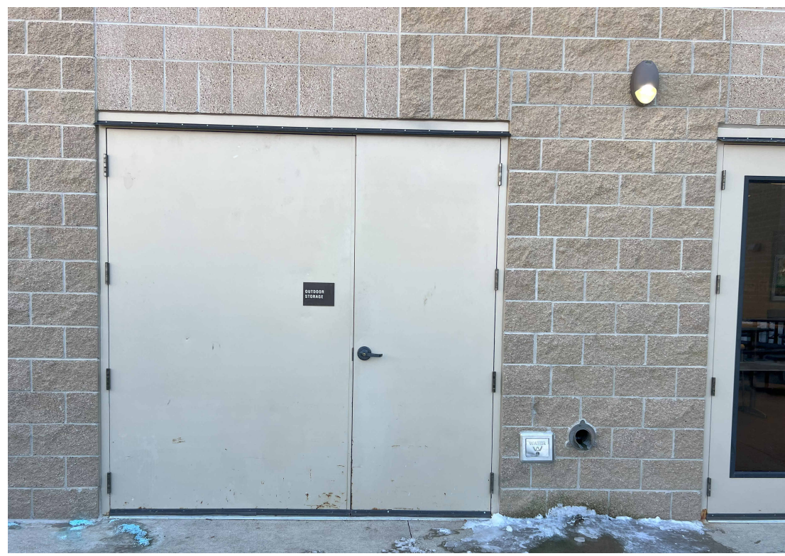
Outside Storage door - Demolition
