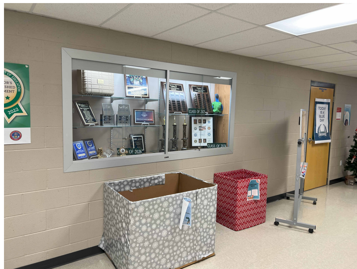
Trophy Case - Demolition
